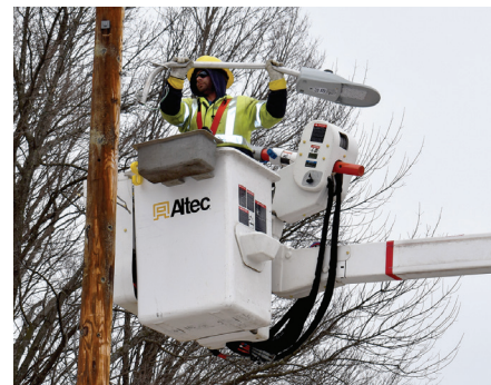
CWEC Service Foreman John Bestul installs a new LED light fixture to a light pole in the village of Tigerton.
